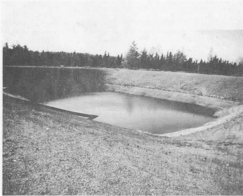
FIGURE 69 Emergency Active Liquid Disposal Pit
